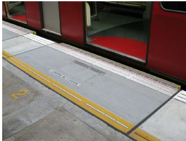
Figure 4: Mechanical gap fillers at EAL Lo Wu Station
