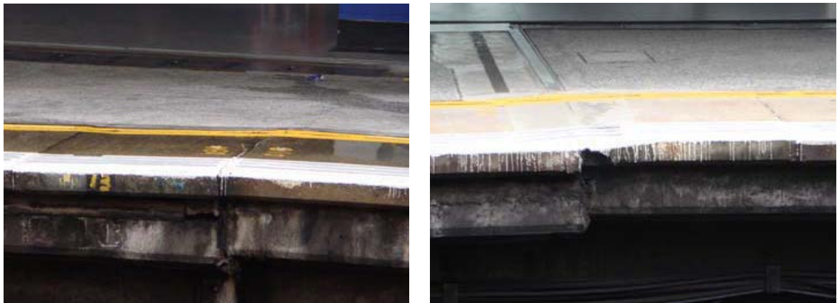
Figure 7: Construction works for platform at EAL stations
