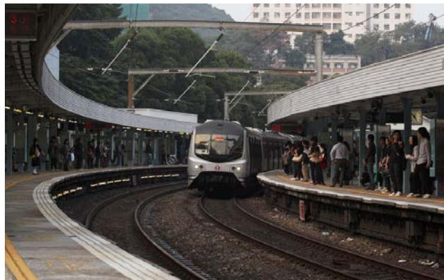
Figure 2: Curved platform at an EAL station
